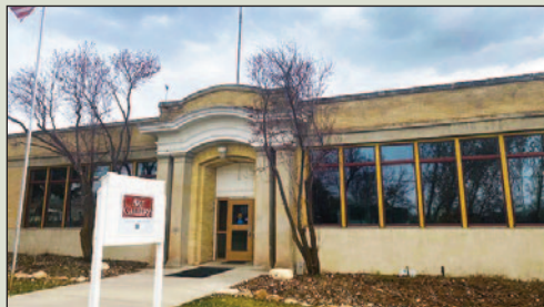
New windows at the Spring City Activity Center.
